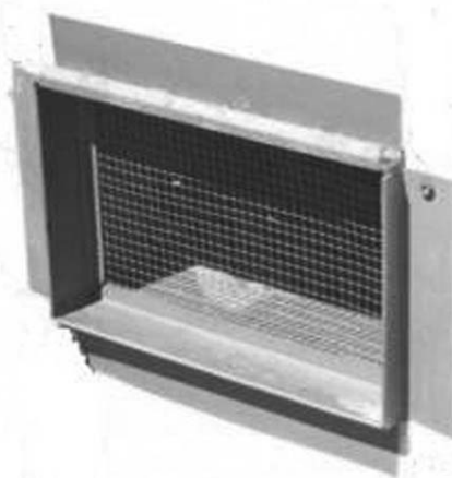
CRAWL SPACE VENT INSTALLED
