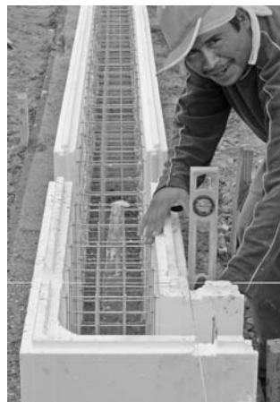
CHECK FOR LEVEL AND PLUMB
