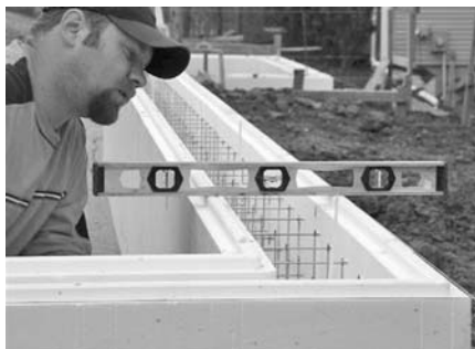
CHECK FOR LEVEL AND PLUMB
