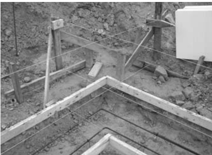
SET BATTER BOARDS AND STRING LINES
