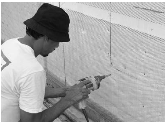
SCREW LATH TO ATTACHMENT STUDS
