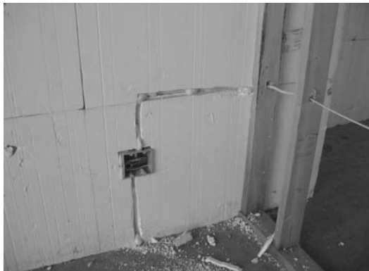
ELECTRICAL BOX & WIRE INSTALLATION
