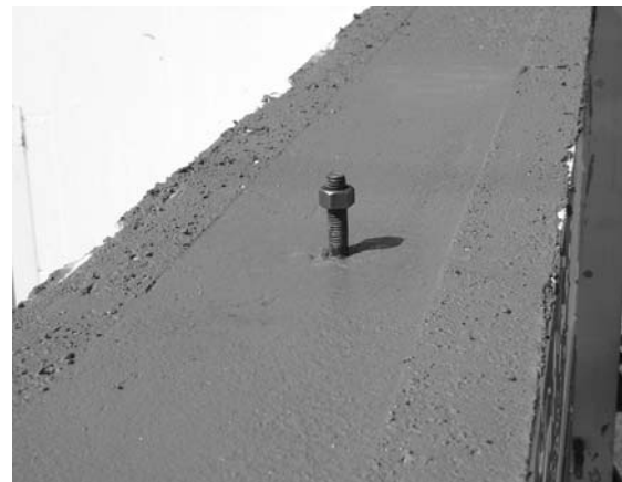
INSTALL ANCHOR BOLTS
