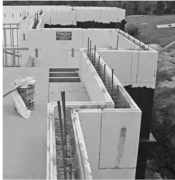
EXTEND REBAR FOR OVERLAP
