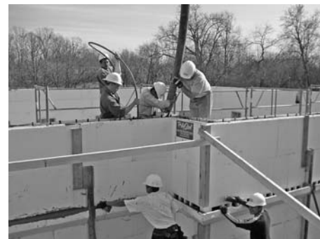
BOOM PUMP PLACEMENT
