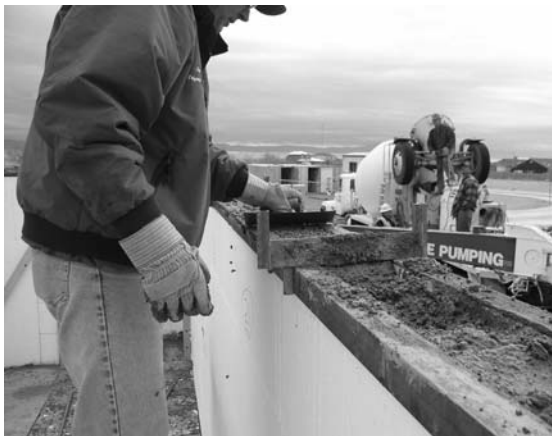
SCREED TOP OF WALL
