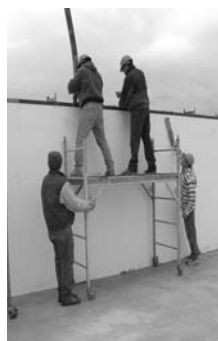
ROLL AROUND SCAFFOLDING
