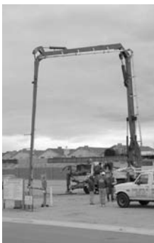
BOOM PUMP WITH REDUCER HOSE
