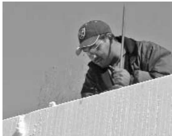
INSTALLING VERTICAL REBAR
