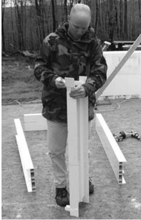
INSERT CORNER CONNECTORS
