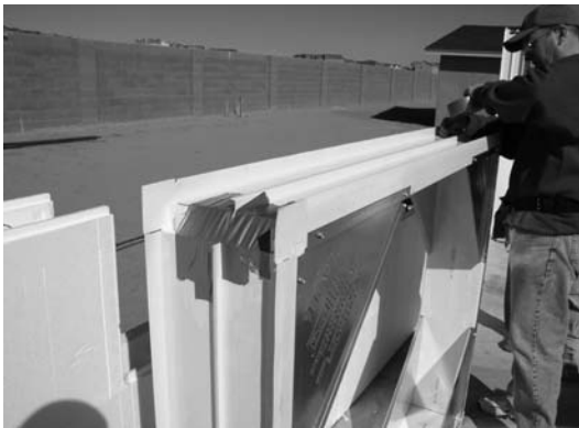
TAPE ENDS TO PREVENT CONCRETE INTRUSION
