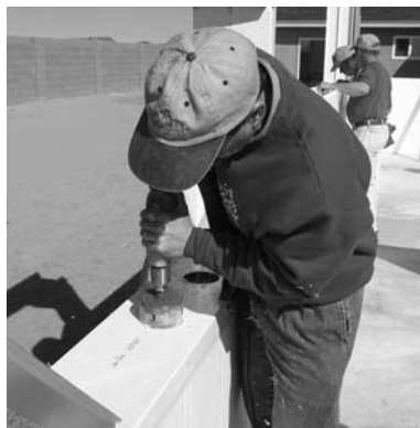
DRILL OR CUT PORTS OR SLOTS
