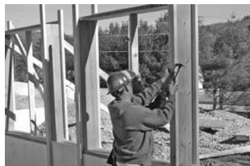
WOOD BUCK INSTALLATION
