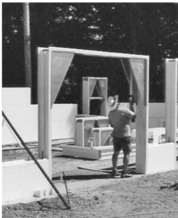
DOOR BUCK INSTALLATION
