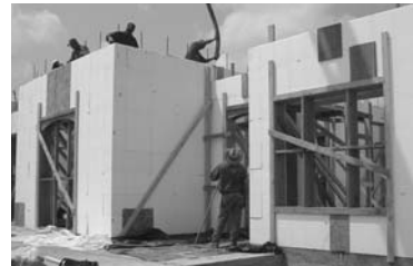
WOOD BUCKS INSTALLED & BRACED
