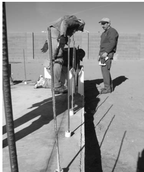
REBAR WITH PVC RINGS
