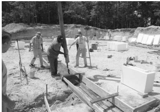
CONSTRUCT A LEVEL FOOTING
