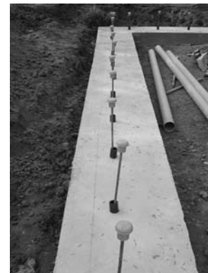
CONSTRUCT A LEVEL FOOTING
