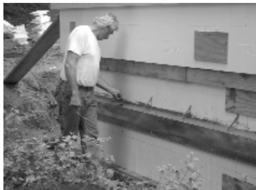
FINISHING METAL BRICK LEDGE
