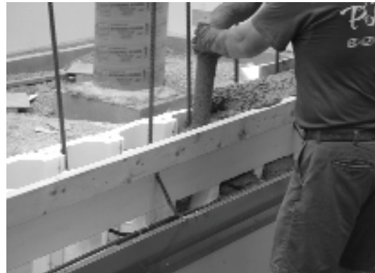
METAL BRICK LEDGE POURED
