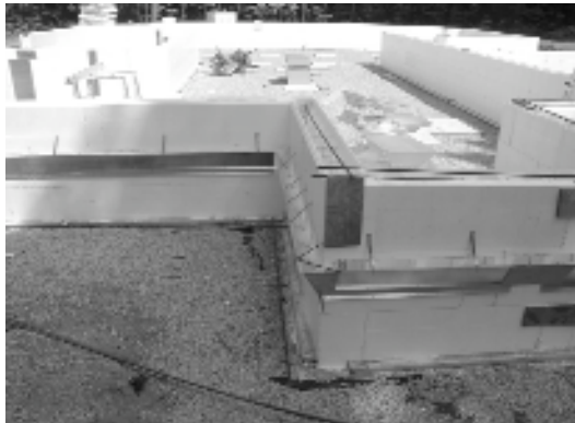
METAL BRICK LEDGE INTALLED
