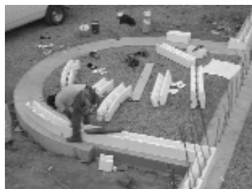
INSTALLING CURVED WALLS
