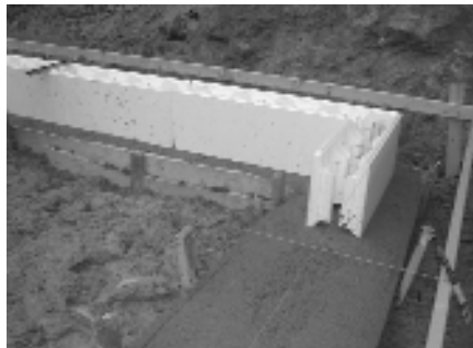
SET BATTER BOARDS AND STRING LINES
