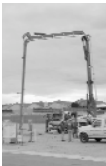
BOOM PUMP WITH REDUCER HOSE
