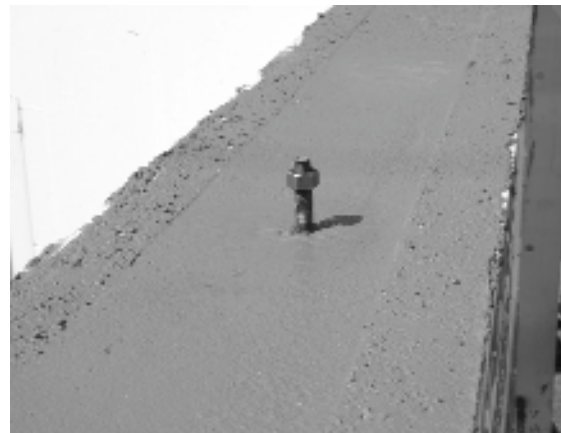
INSTALL ANCHOR BOLTS
