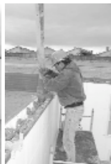
BOOM PUMP PLACEMENT
