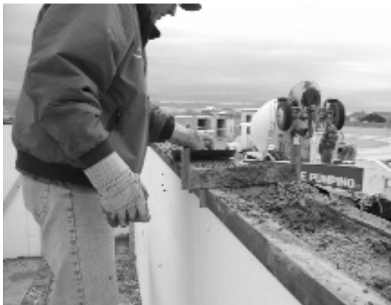
SCREED TOP OF WALL
