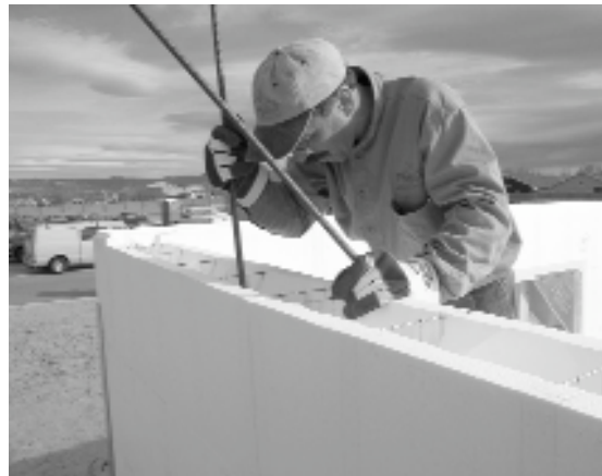
INSTALLING VERTICAL REBAR
