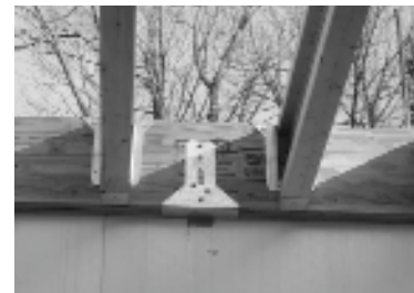
SIMPSON HANGER WOOD LEDGER INSTALLED
