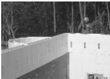
SIMPSON HANGERS INSTALLED
